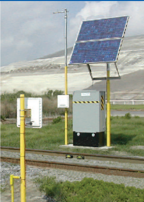
Remote site utilizing solar power and RF communications
